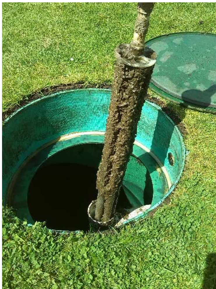
Figure 2 Blocked filter
